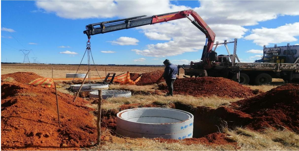
Figure 3: Fitting of concrete rings into excavations.
